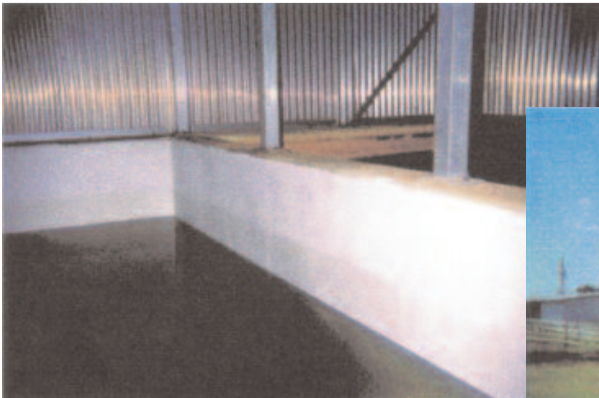
Interior view of the treated water holding tank completed with Sider-Proof FF-PR Coating
